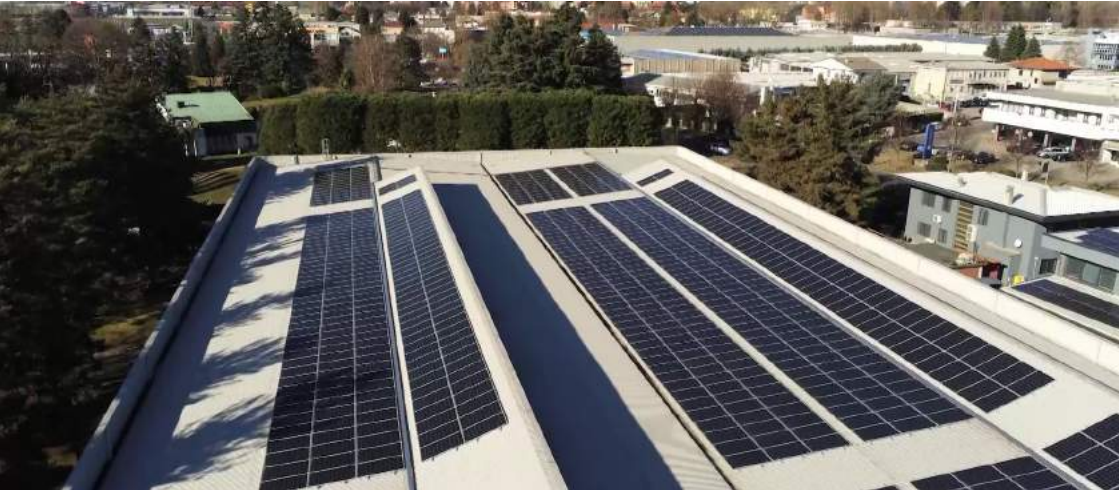
Photovoltaic system of Saronno factory. Power: 400 kWh
